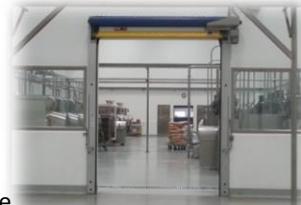
[2nd Mixing Room]
